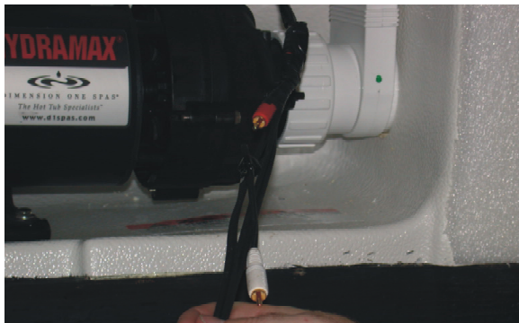
Figure 15. Attaching Cables and Harness to Fish Tape
